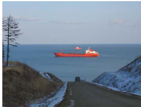
Tanker Loading Facility
