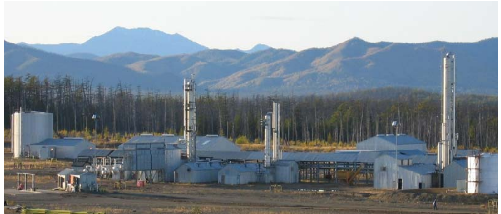
Refinery and Refined Product Storage
