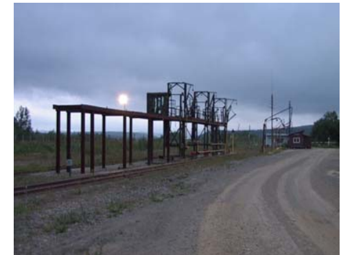
Rail Loading Rack
