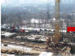
Zapovednaya, bldg 5, April 2010
