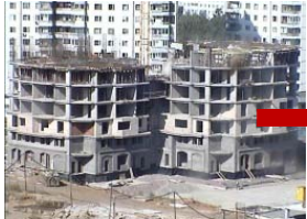
Ak, Vinogradova, bldg 7, August 2009
