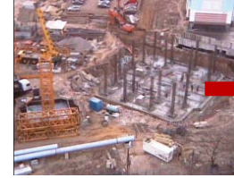
Zapovednaya, bldg 6, April 2010
