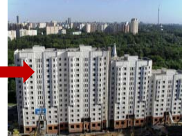
Zapovednaya, bldg 5, September 2010
