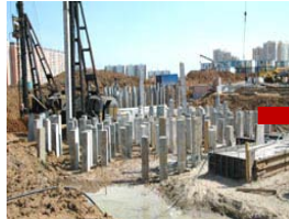
Novokurkino, Khimki, bldg 21 March 2010
